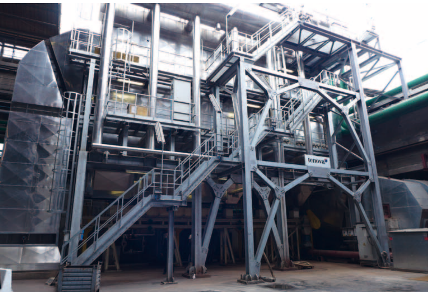
Fig. 5 - The new iRecovery system, heat recovery section.
