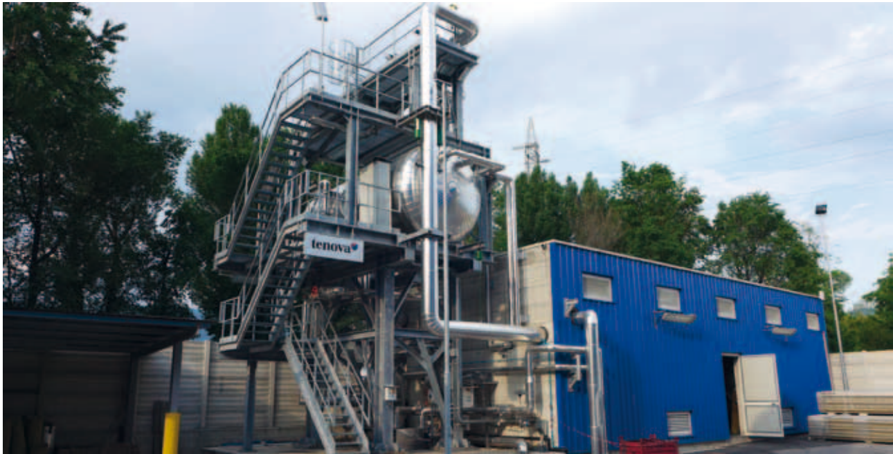
Fig. 6 - The new iRecovery system, A2A exchange section.
