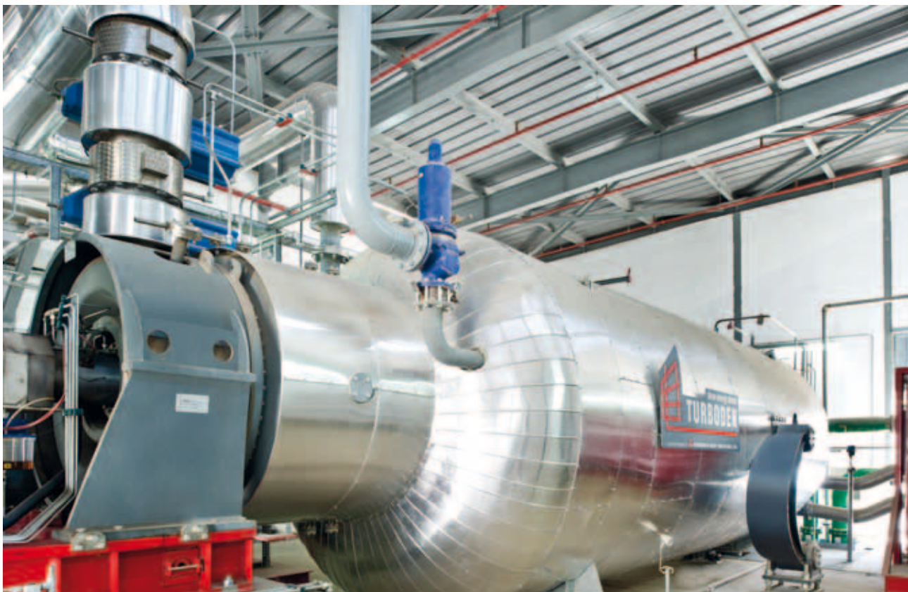
Fig. 7 - The ORC turbo-generator (by courtesy of Turboden).
